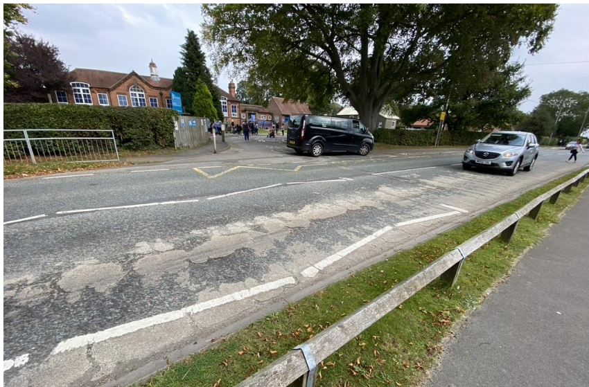
A view showing the deterioration of the road surface and markings in front of the school.
