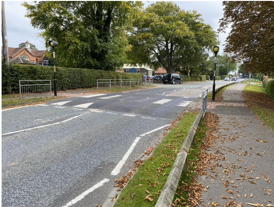
A view showing the deterioration of the road surface and markings in front of the school.
